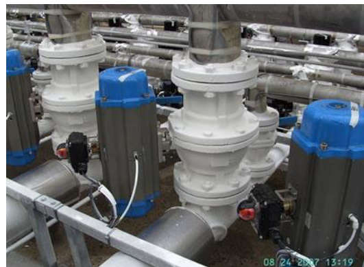
Shows reduction to 29°C after application of industrial insulation coating
