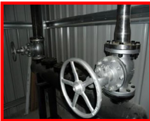
Pipework Prior to Application
