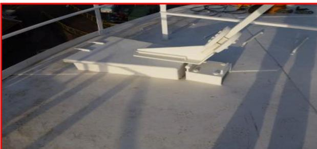
The energy retention capabilities of Mascoat Industrial Insulation (DTI) make it a popular choice for insulation among the oil and gas companies internationally. Inspectability of the tank surface is often a factor that is not provided with most conventional insulation. The thin coating of Mascoat DTI allows full inspectability and the ability for personnel to also walk on coated surfaces safely.
